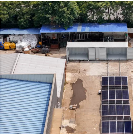
modular building solar system
