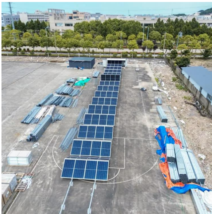
Energy storage container, BESS container
